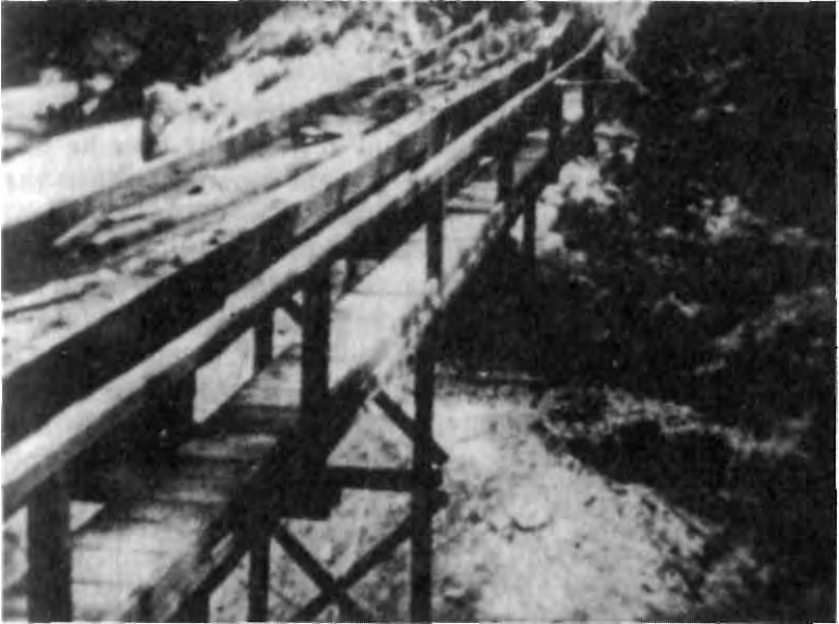
Logging Flumes in Neuburg.
