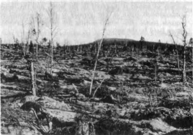
Preparation of ground surface after felling by the Deman works in the Gallivare region (Pal-Nils Nilsson/Trio).
