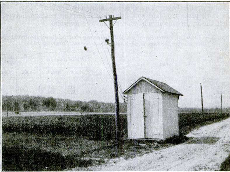
FIG. 1.—General view of the experimental field at Arlington Experiment Farm, showing the system of double insulators used in suspending the wire network from poles and the power lines leading to the motor in the apparatus house (foreground). Poles supporting the grounded network along the side of the control plat may be seen in the distance. (Photographed May 8, 1913.)
